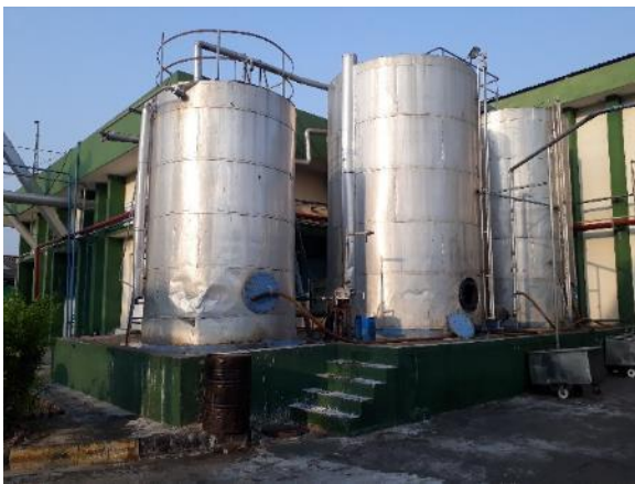
Tallow Chamber used for storage of fats
